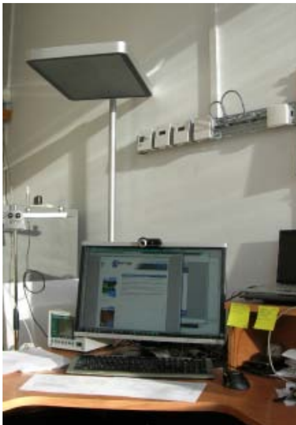
Figure 7. Left: Wall-mounted IAQ-modules for ventilation control and dimmable lighting at the test building in Prague. Right: Web-based monitoring system with room probes for IAQ, temperature, relative humidity and illuminance measurement using the normal UTP infrastructure of the building. The FlexProbe serves as interface hardware between room probes and software.
