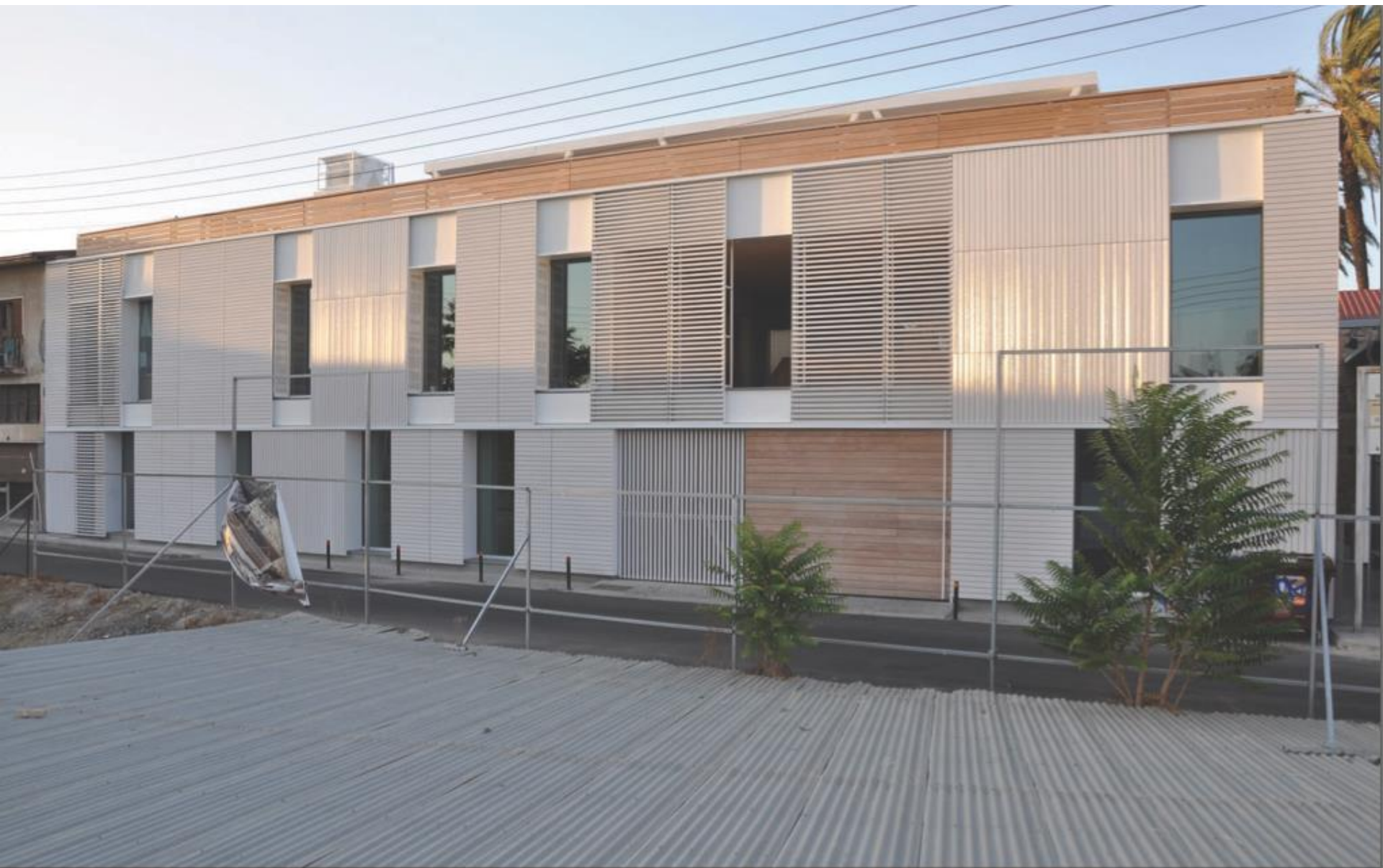
Nicosia Municipality. Finance Department - South Facade
