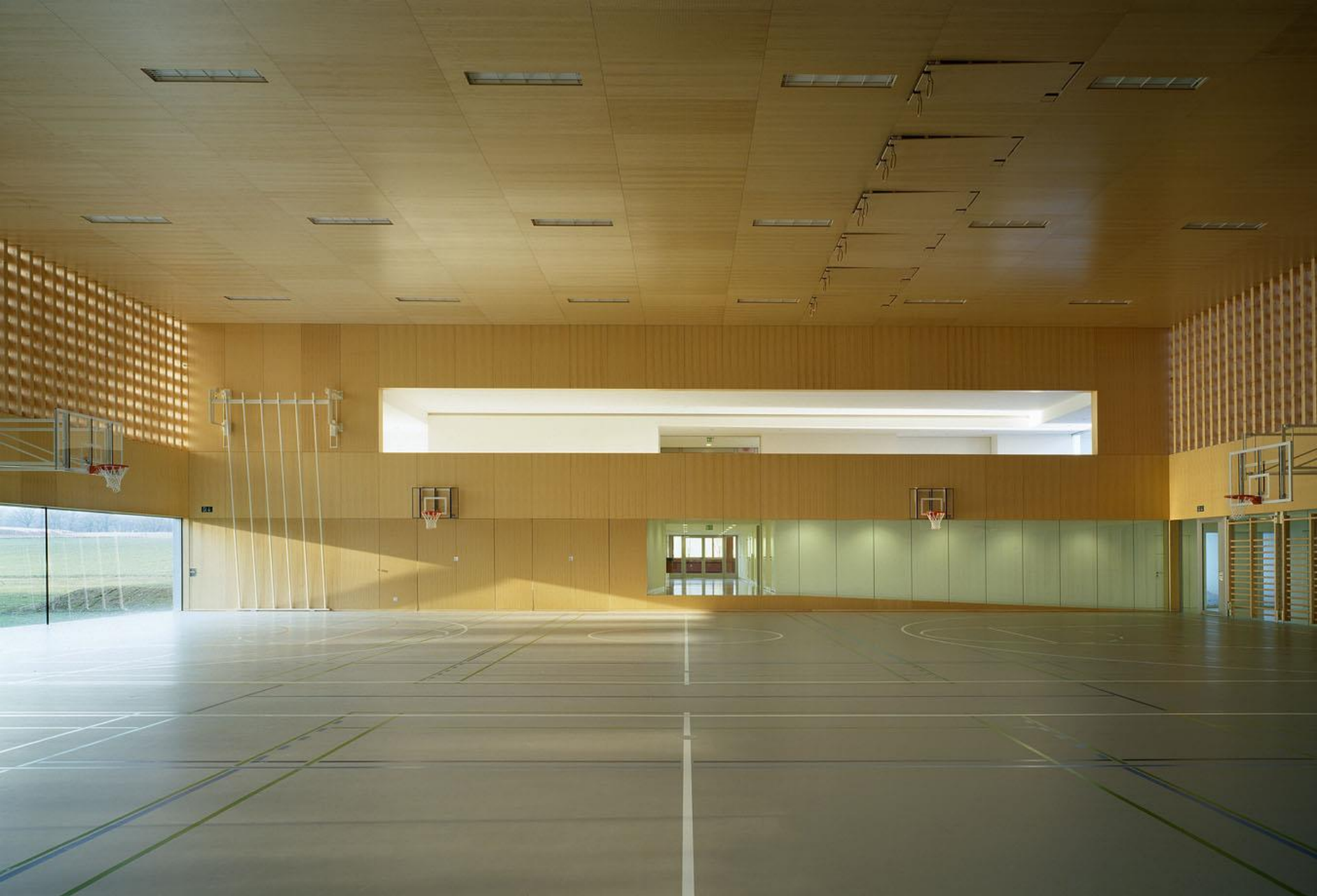
the ventilation inlet grid / storage room door
