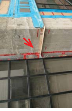
Figure 28: Overall view of the interface detail in figure 27 after removing the adjacent masonry.
