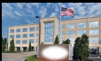
Duluth, GA; Climate Zone 3A LEED Gold
