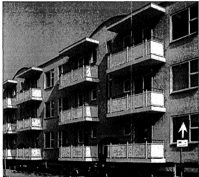
Figure 2: There are more financial means for retrofitting. In this project in Hengelo the Netherlands, completely new facades and MFAs (multifunctional appliances) were applied
