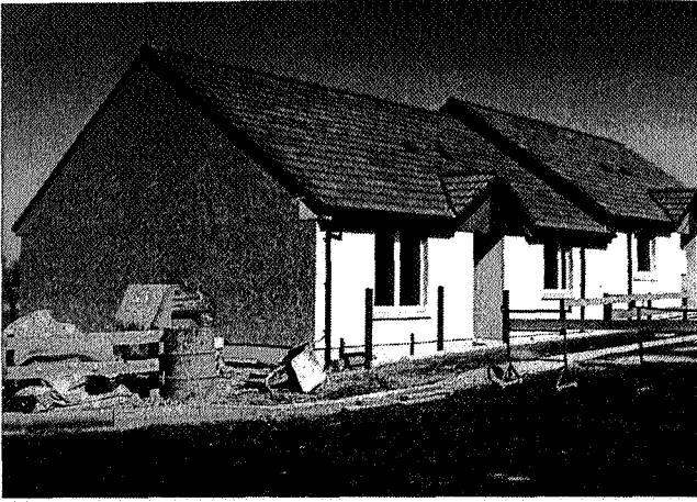
Figure 1 The low energy houses (UK Crown Copyright 1994)
