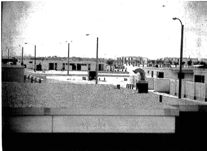
Figure 4 - The horizontal spread is illustrated for this single-story housing located in the Middle East. Cooling is supplied by a central chiller plant. Gooseneck kitchen exhausts are one point of air infiltration.
