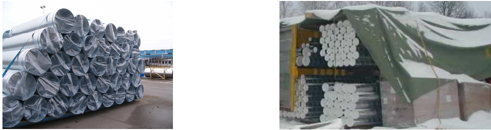
Figure 5. According to the Finnish Classification for indoor environment the ducts and components need to be protected during transportation and storage.
