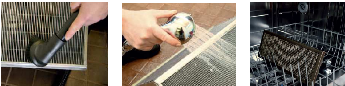
Figure 7. Cleaning instructions for heat recovery coil and kitchen extract filter.
