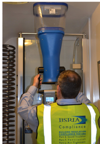
Figure 3: Assessment of ventilation system performance using a powered flow hood
