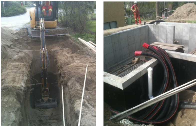
Figure Four: Trenching and laying earth tubes for case study project
