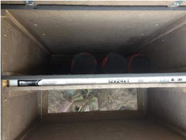
Figure Six: Air inlet with screen, mesh and filter – all upstream of the earth tubes.
