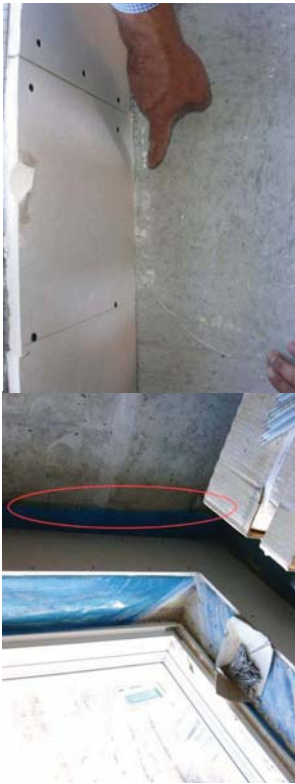
Figure 6. Left: Correct connection with overlap; Right: Missing overlap
