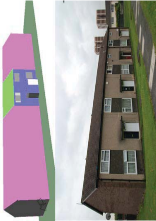
Figure 6. Case study of the mid-terraced house in Leeds and the model built in IES VE.
