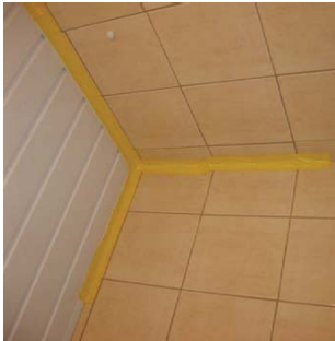
Figure. 2. The examples of leakages in the walls and ceiling of the apartments
