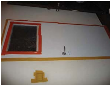
Figure. 3. Method of sealing of bathroom's door in the flat of the 11-storey building
