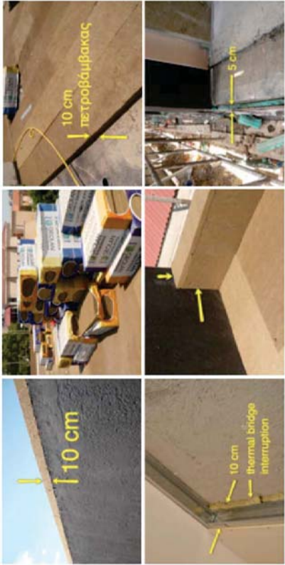
Figure 4. Outside thermal insulation with minimised thermal bridges is composed mostly by 10 cm rockwool. Foundations are insulated with 5 cm xps. In some special cases it was necessary to use internal thermal insulation with 10 cm rockwool.
