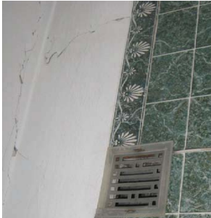
Figure. 2. The examples of leakages in the walls and ceiling of the apartments
