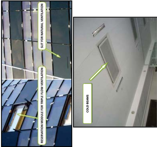
Figure 5. Air distribution principle
