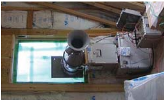
Figure 2. Measuring air tightness.
