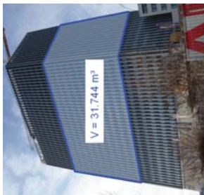
Figure 4. BlowerDoor test in the marked part of this high-rise building
