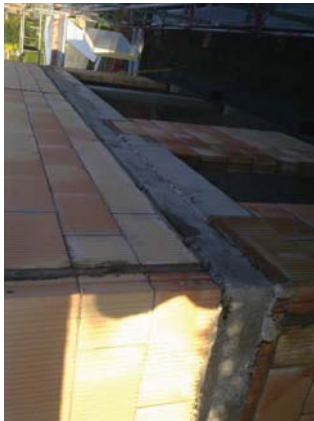
Figure 10: The ends of the hollow core slabs have been filled with concrete
