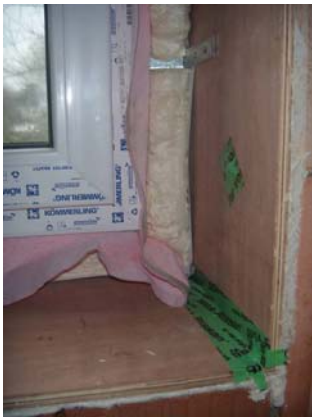
Figure 9: Insulation and installation of the windows
