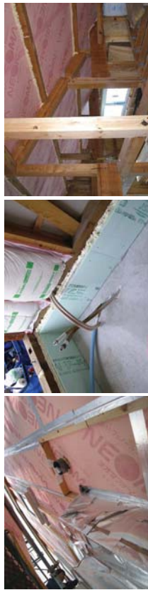
Figure 3. Examples of airtight construction methods. (Left:house_A, Middle:house_B, Right:house_C)
