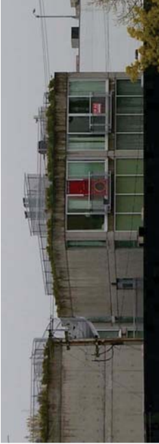
Figure 2. Test Building: the fan setup is visible in the balcony door of unit 611/610 (above). The test fan was always on the Leeward side of the building.
