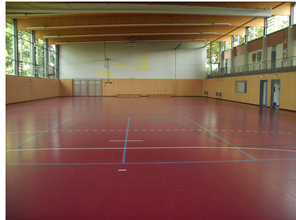
Figure 3: Picture of the sports hall in Sontheim giving an overview of the geometry
