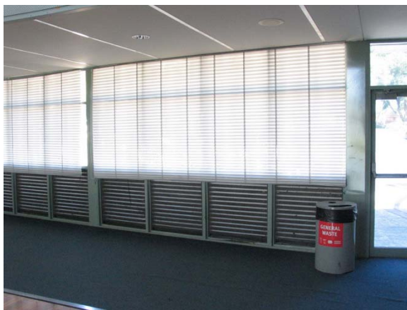
Figure 2 : Open vent along the west wall
