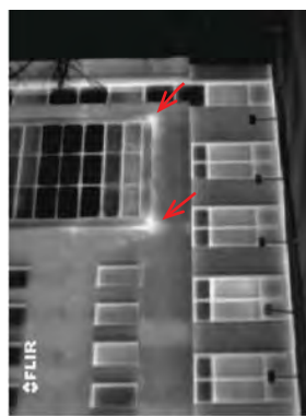
Figure 4: Conductive heat loss at masonry structural shelf angle support (building under positive pressure).
