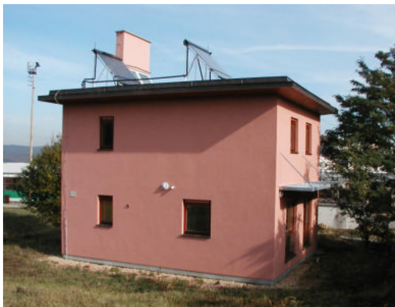
Fig. 12 Demonstration house with hybrid ventilation
