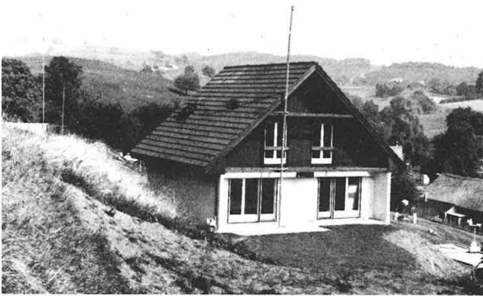
Plate 1: View of test building from the West
