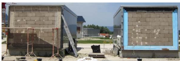
Figure 1 : Passys cells with hempcrete walls
