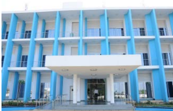
Figure 12: The north façade and building entrance.
