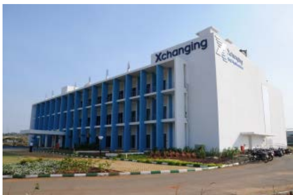
Figure 13: The completed building (from northwest)
